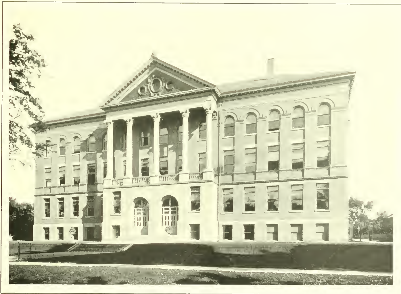
UTICA FREE ACADEMY — KEMBLE STREET Completed 1890, at a cost of $135,000 — The building is 140 x 181 feet, and has capacity for 850 pupils
